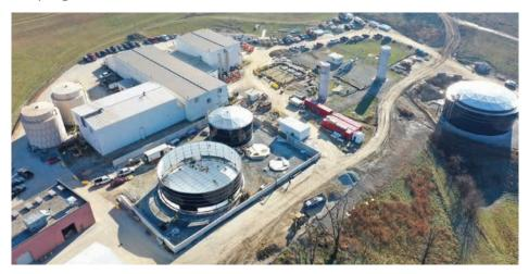
To meet ever-more stringent state and federal standards, these latest upgrades include installation of massive water storage tanks (pictured above) and advanced reverse osmosis technology that will greatly enhance the plant's performance and enable the facility to meet new permit requirements.
